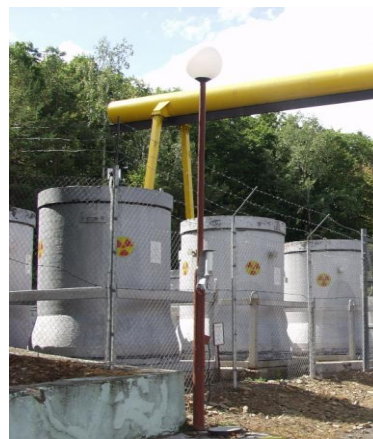
Fig.24 A set of concrete containers type "GOU." Used for storage of spent gamma irradiation devices
