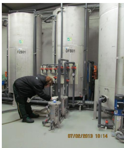
Fig.6 Columns for purification of LRAW
