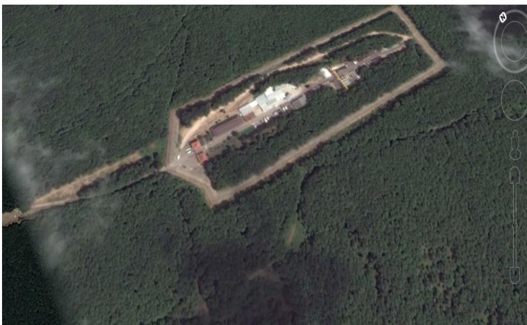
Fig. 2. View of the site
