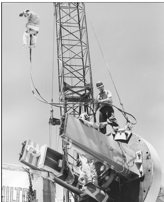
Figure 4. Super Kukla reactor during installation
