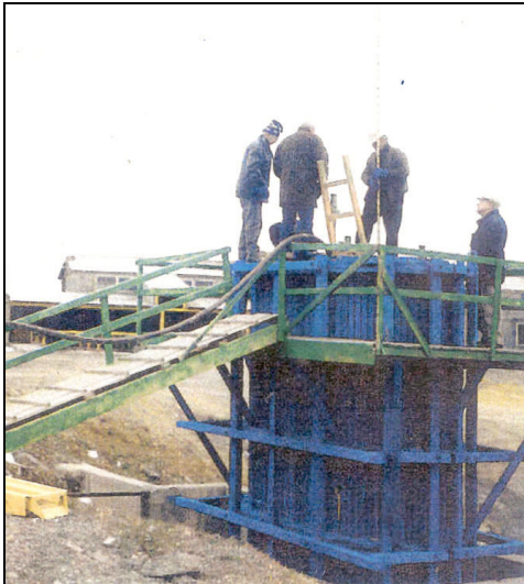
Figure 6. Georgia IRT Mockup for reactor grouting
