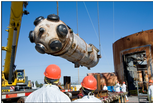
Figure 1. Removal of HWCTR Steam Generator.
