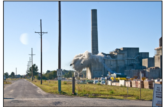
Figure 5. Demolition of P reactor stack.
