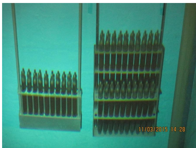
Fig.2 Irradiated fuel rods kept in the pond of TINT 2 MW Research Reactor
