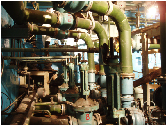
Figure 2. General view of the PCC pipe-lines
