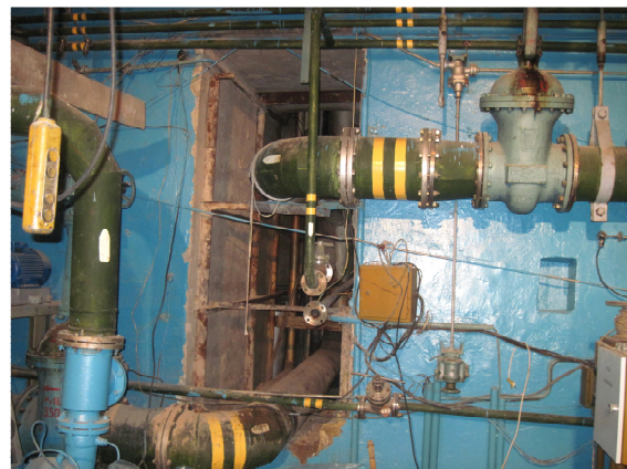
Figure 5. Window in the concrete wall.
